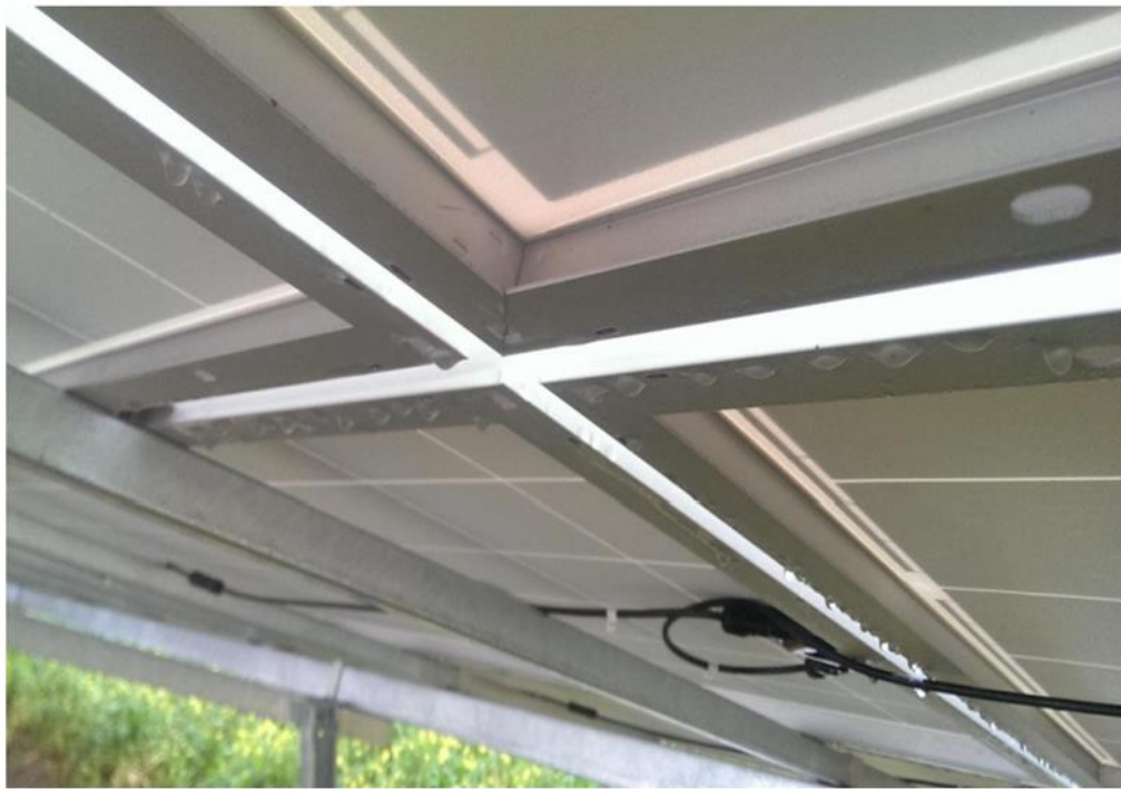
Figure 7. Underside of a solar panel
